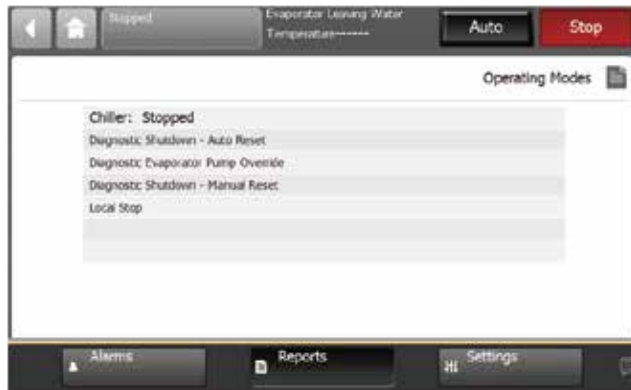
Figure 43. Chiller Operating Modes screen
