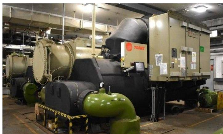
Following the commissioning of the newly installed CenTraVac™ chillers at the QGO in 2021, the building's HVAC system has seen a significant increase in operating efficiency, which helped achieve an energy saving of over 30 percent and a carbon emission reduction of over 900 tonnes per year.
