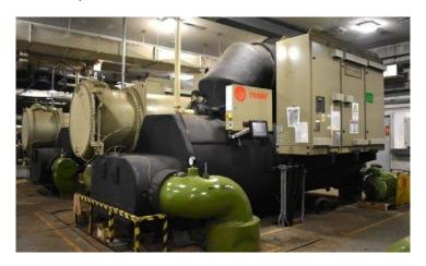
Following the commissioning of the newly installed CenTraVac<sup>™</sup> chillers at the QGO in 2021, the building's HVAC system has seen a significant increase in operating efficiency, which helped achieve an energy saving of over 30 percent and a carbon emission reduction of over 900 tonnes per year.
